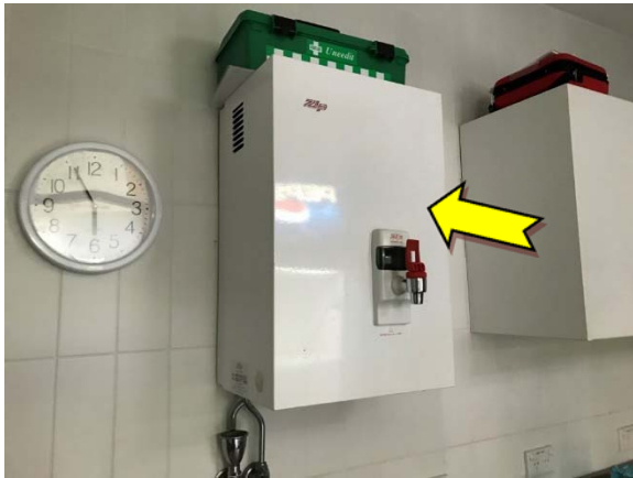
Photo 3. Exterior, west elevation, hot water heater – suspected SMF internal insulation.
